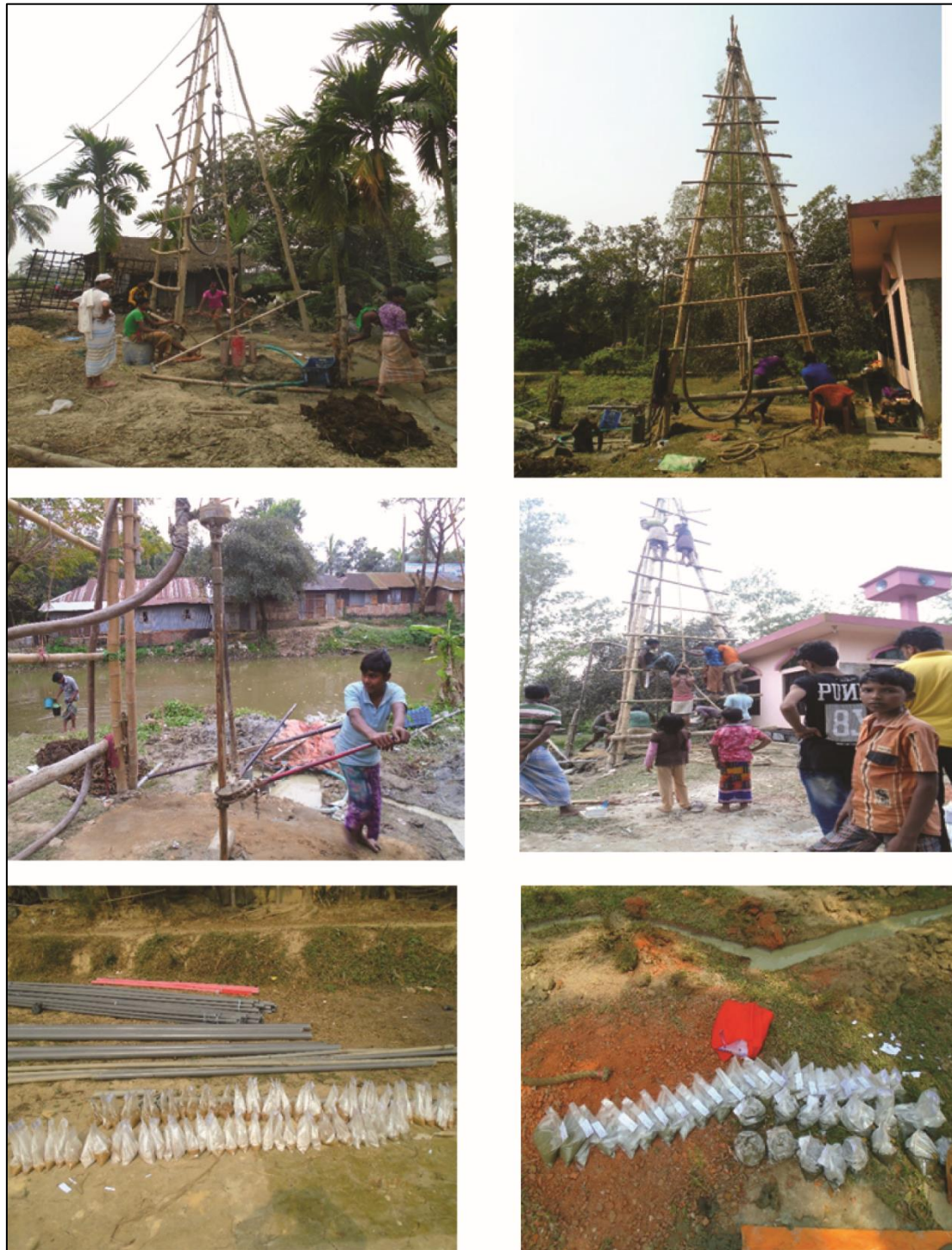
Figure 3: Monitoring well drilling and Wash samples.
