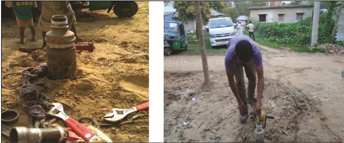
Figure 4: Established Monitoring well with 3 Inches Housing Pipe.
