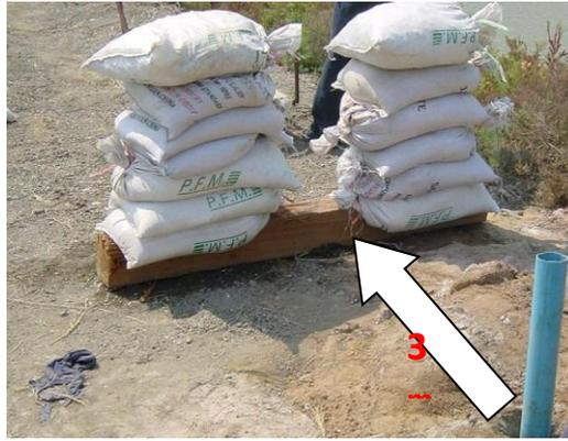
**Figure 2.5 To set the wooden plank and sand bag 3.0 meters from a borehole**
